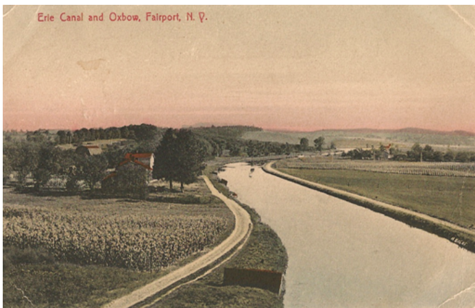
The Oxbow circa 1900 looking south and west from the old Fullamtown Bridge. The site of the 1871 canal break would have been around the middle of this picture to the right.
