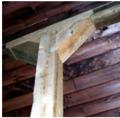
Support structure added to the barn's interior at 8 West Street
