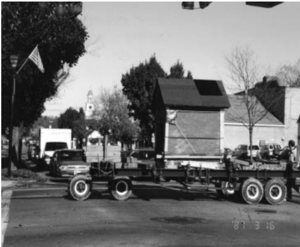
Brick outhouse at the intersection of Main and Church Street being moved to its final destination behind the Potter Memorial Building.
